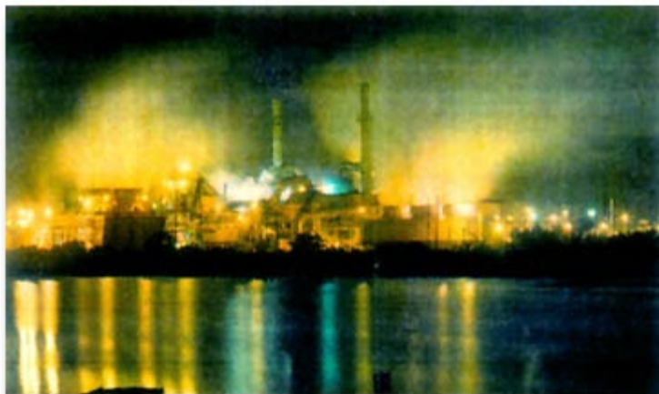
A fertilizer plant where fluorosilicic acid is a most toxic waste by-product produced from the manufacture of phosphate fertilizers.
